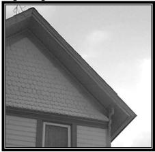
**#Square-cut eave - Soffit is parallel to the roof slope and fascia is** perpendicular with a vertical fascia
